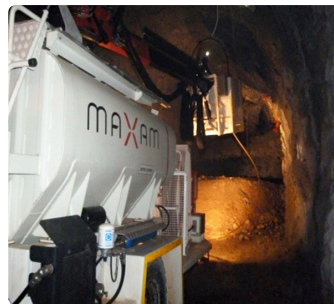
2. RIOFLEX RAPID underground application.
